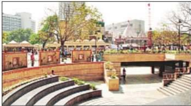
After the upliftment, the Hanuman Vatika now has proper walkways, public conveniences and seating arrangement. HT PHOTO
